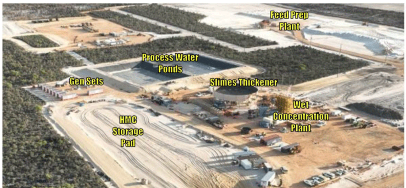
Photo 1 - Atlas Project Construction Progress - 31 December 2024
