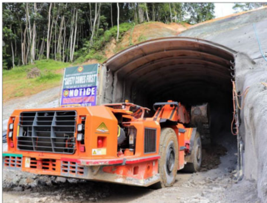
Photo 1: View of the portal area for the Tigerway Decline Portal.
