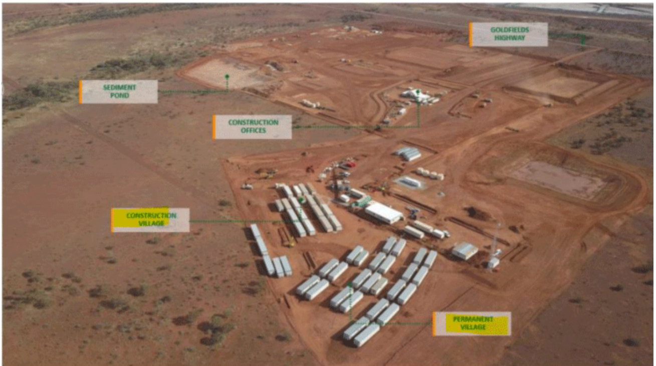
Figure 2: Accommodation village and process plant site
